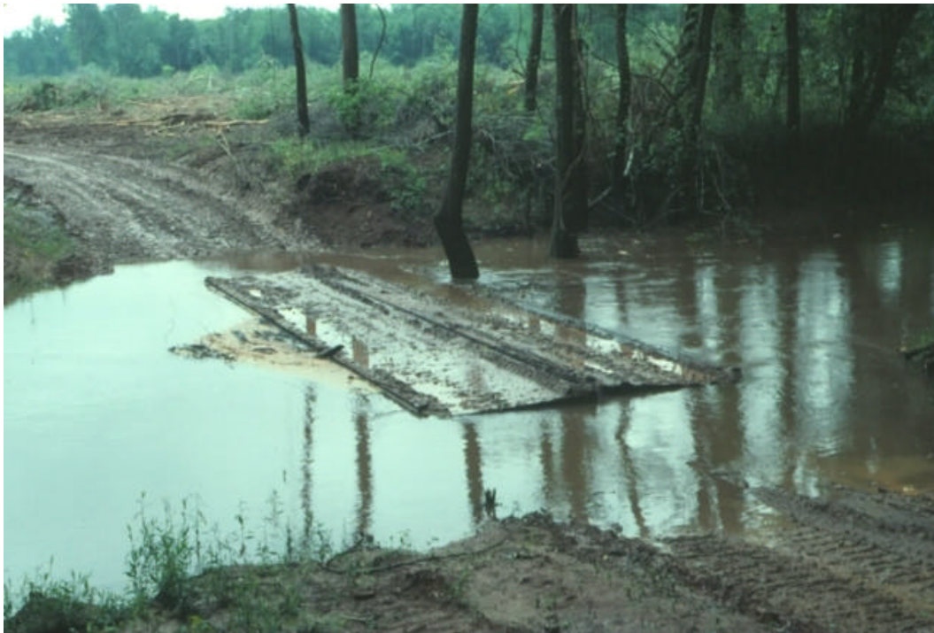
Figure 21. Georgia Pacific bridge in early stages of flood. This photograph illustrates the importance of securing the bridge to nearby trees.
