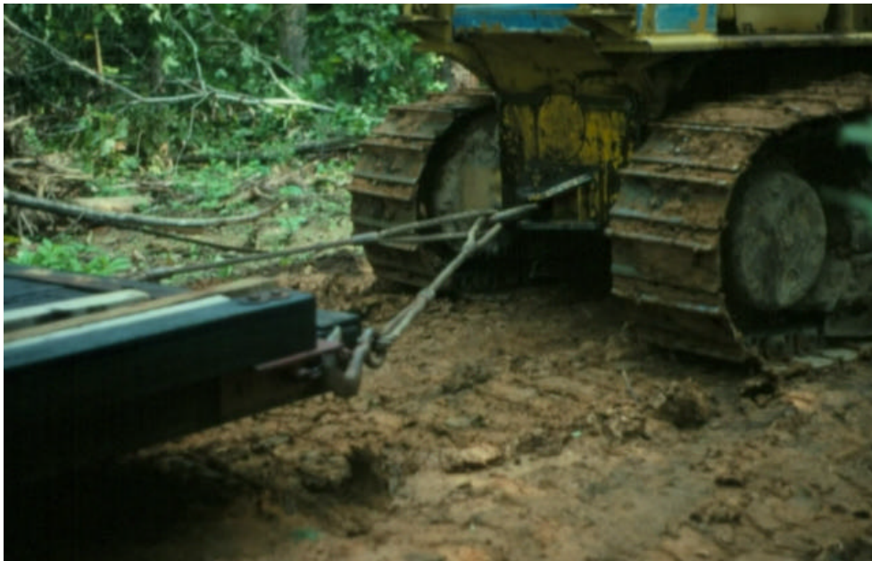
Figure 8. Bridge modules can be skidded short distances to the site using typical construction equipment.
