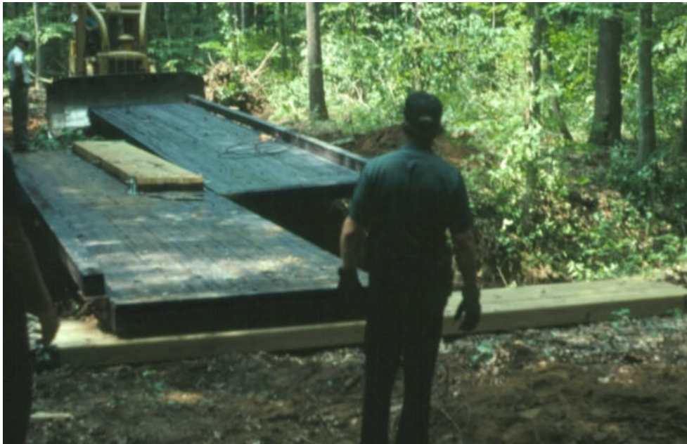
Figure 9. The Morgan County bridge module is being pushed into place by a crawler tractor.
