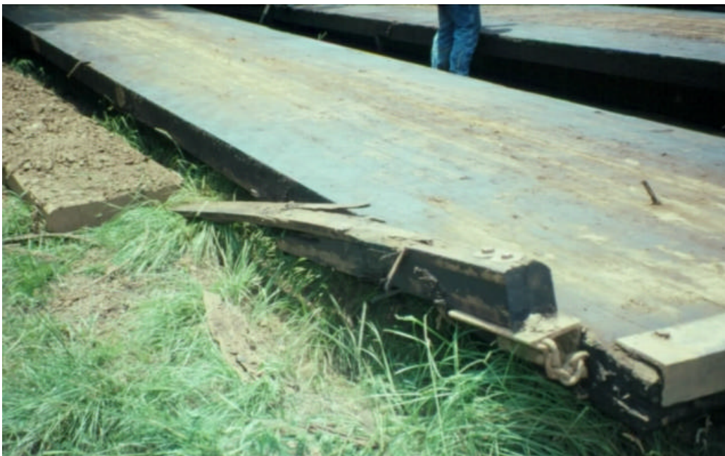
Figure 23. Broken curb rail on the Georgia Pacific bridge after a removal by a grapple skidder.
