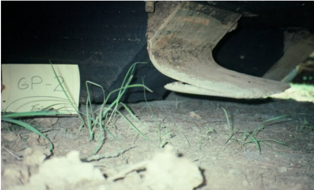
Figure 24. Bent steel protector plates on the webs of the Georgia Pacific bridge after skidding a long distance over a gravel road.
