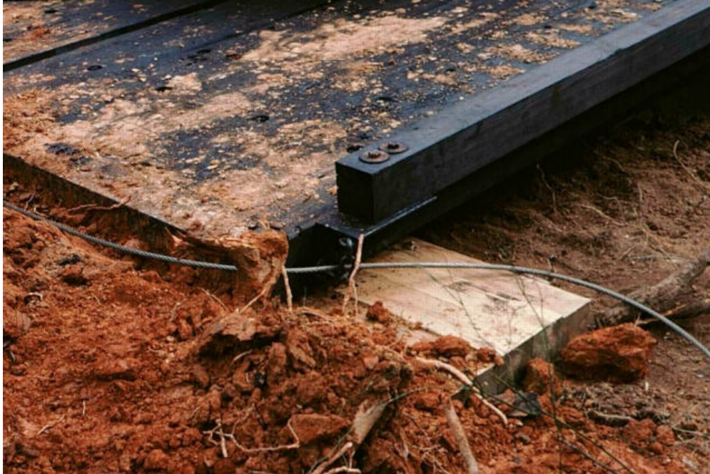
Figure 5. Curb rails and steel hardware on the finished T-section bridge module.
