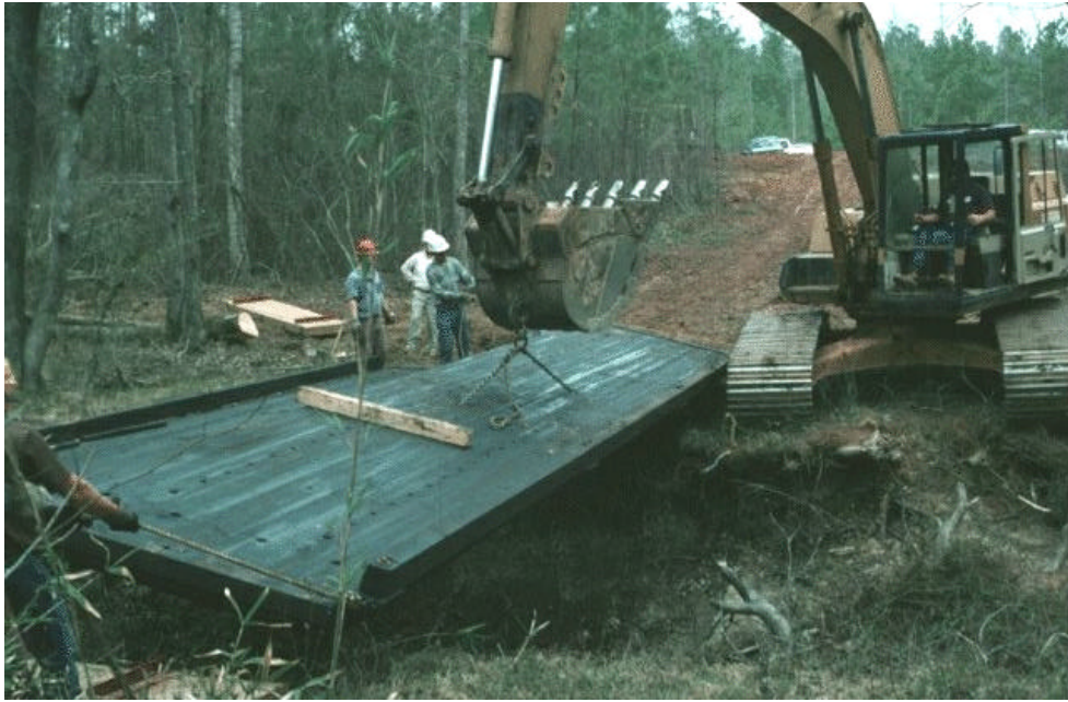
Figure 7. Installation of a bridge module using a typical excavator.
