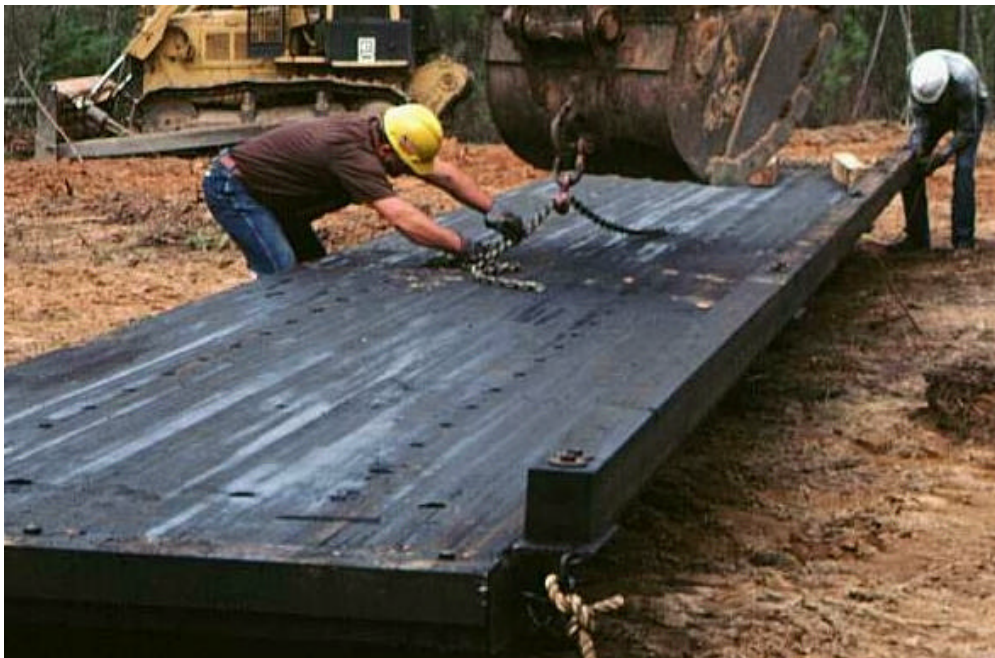
Figure 6. Workers place chains through the steel reinforced lifting eyes before moving the bridge module.
