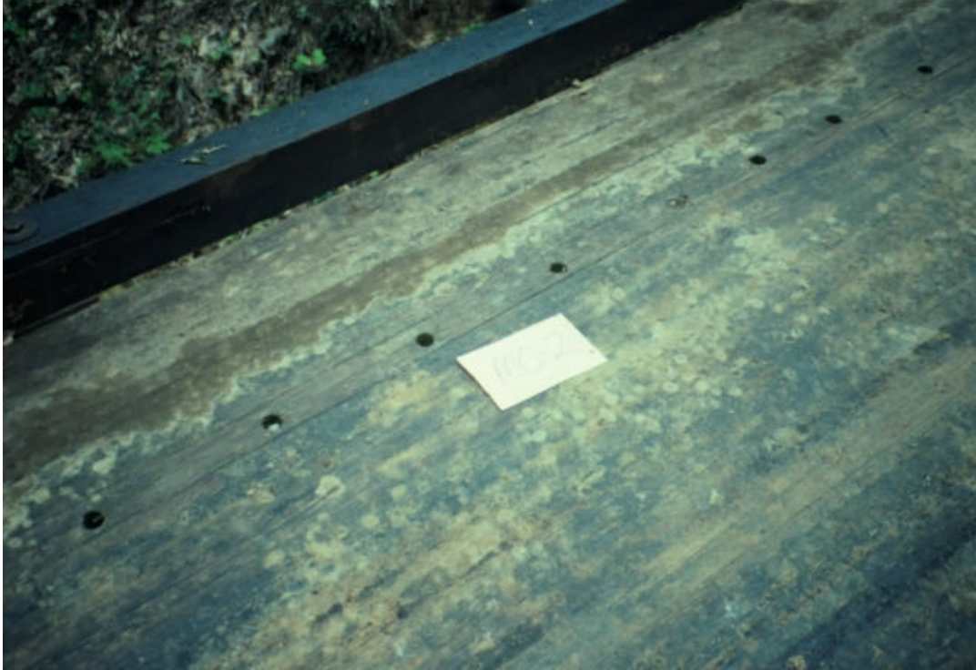
Figure 26. Checks in the top surface of the flange of the Morgan County bridge.
