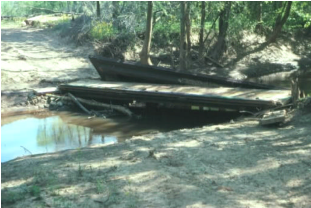
Figure 22. Georgia Pacific bridge after floodwaters had receded. The bridge was subsequently repositioned and the timber harvesting operation was completed.
