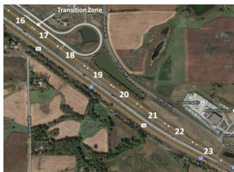
Figure 1. Figure 1. (a) Aerial view of MnROAD Cracking Sections on MnROAD Mainline, and (b) Section Pavement System Structural Designs
