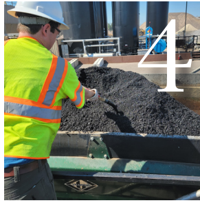
MnROAD Additive Group Test Section Construction
