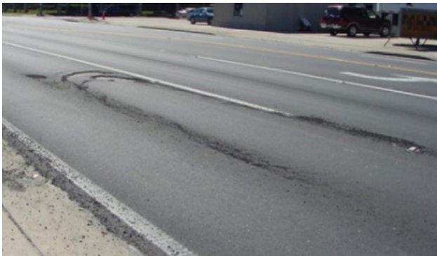
Slippage Cracking
