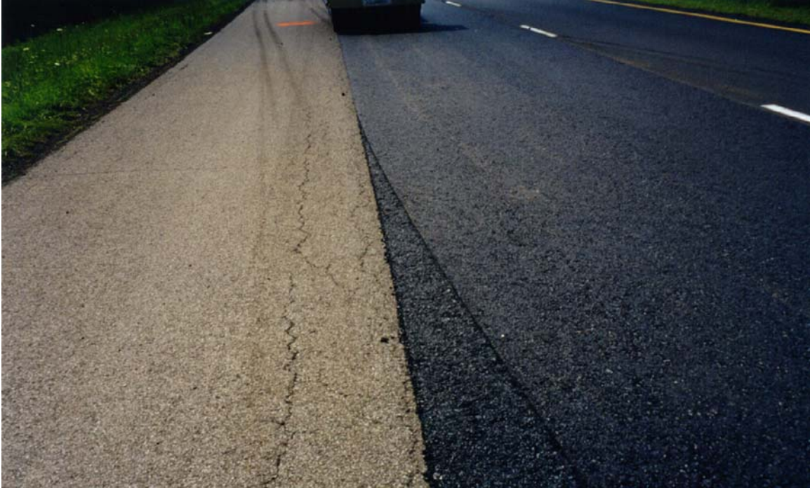
Figure 5. Pavement Surface After One Pass of Breakdown Roller (Roller Mark)
