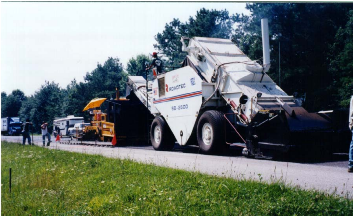
Figure 2. MTV Used on Project
