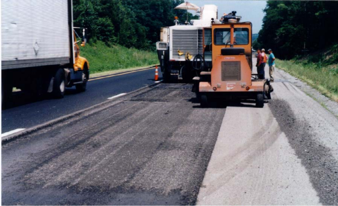
Figure 1. Milling Machine and Sweeper
