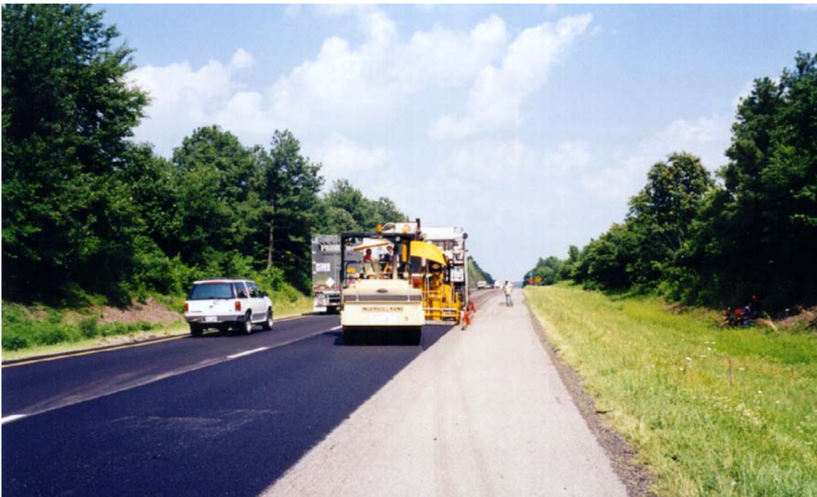
Figure 4. Breakdown Roller
