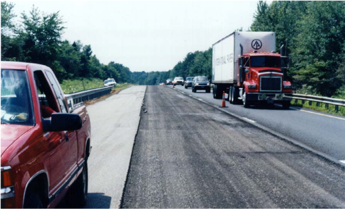
Figure 8. Milled Roadway Showing Vertical Sides
