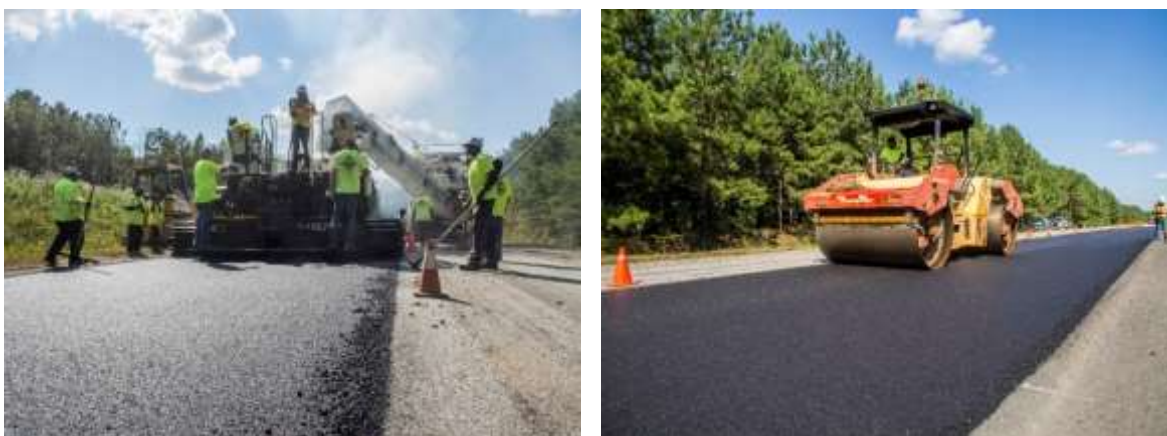
FIGURE 4 Laydown and compaction of S1 surface mix.
