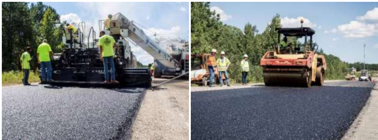
FIGURE 4. Constructing Section S10 with a BMD mix.
