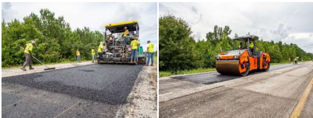
FIGURE 6 Construction of Section S7B.
