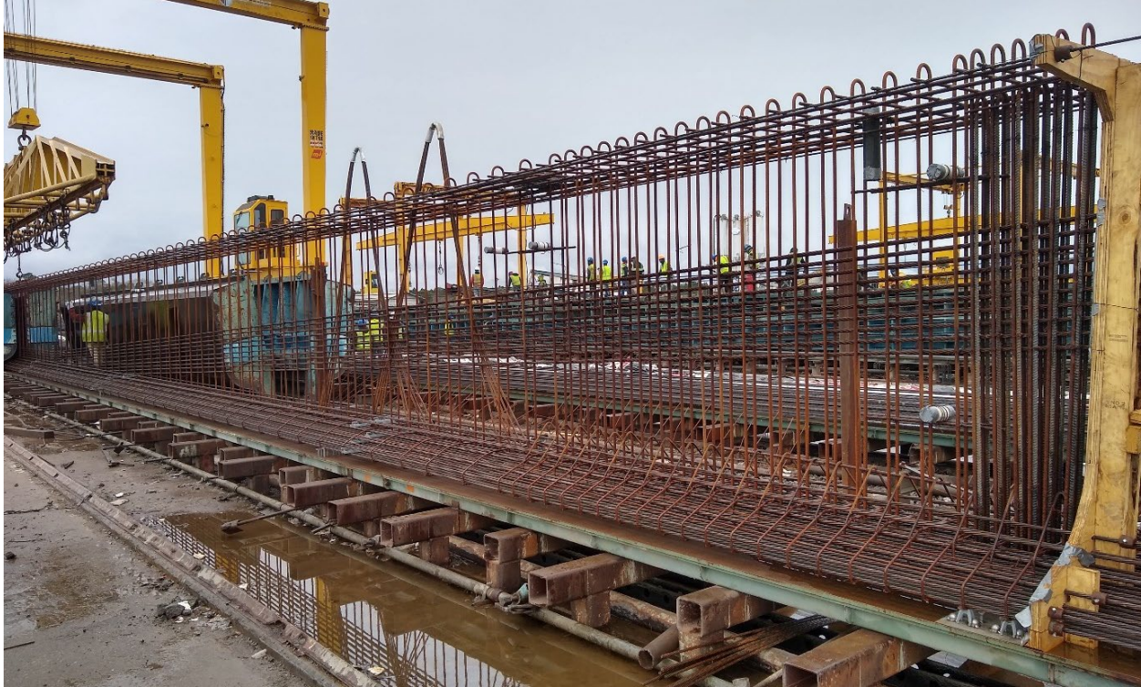
Figure 1-2 WWR reinforcement installed in prestressed girder prior to concrete placement
