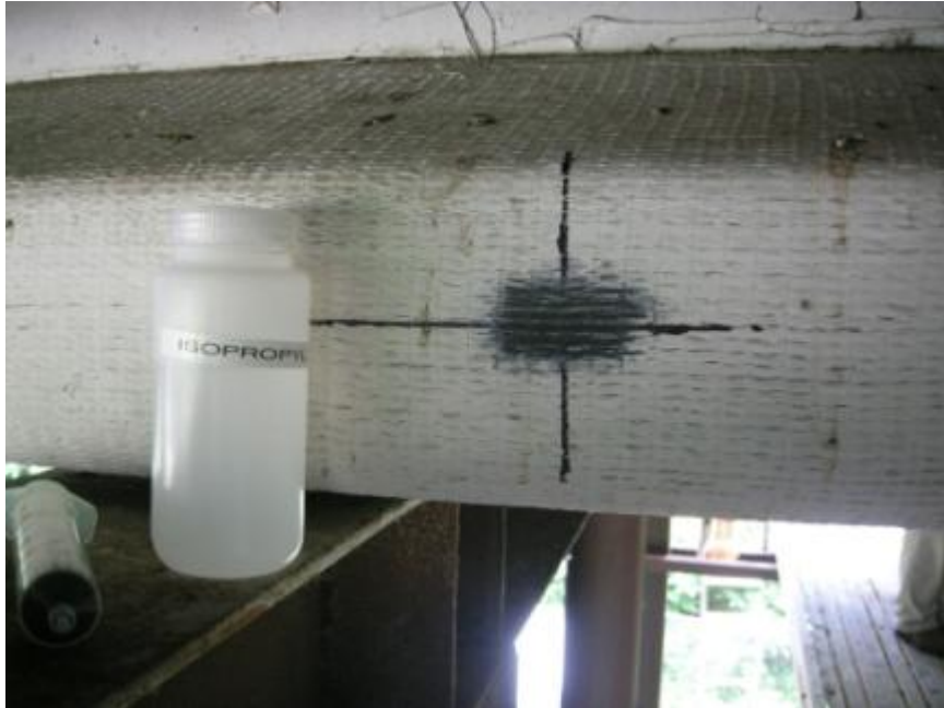
Figure 3.27: Strain gage installation—initial surface cleaning
