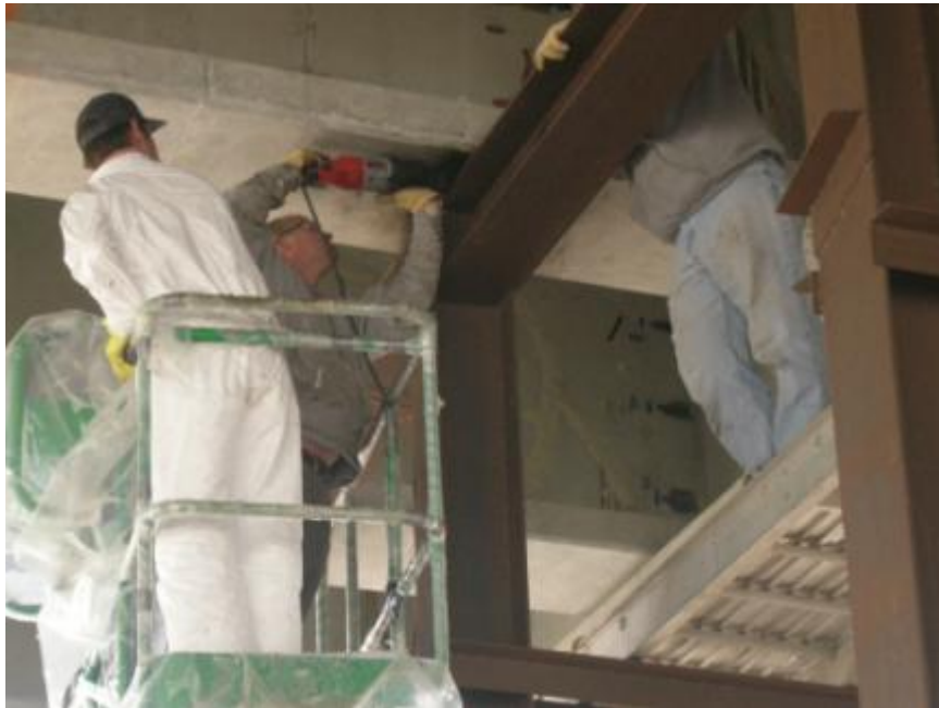
Figure 2.30: Use of saw for bearing pad removal
