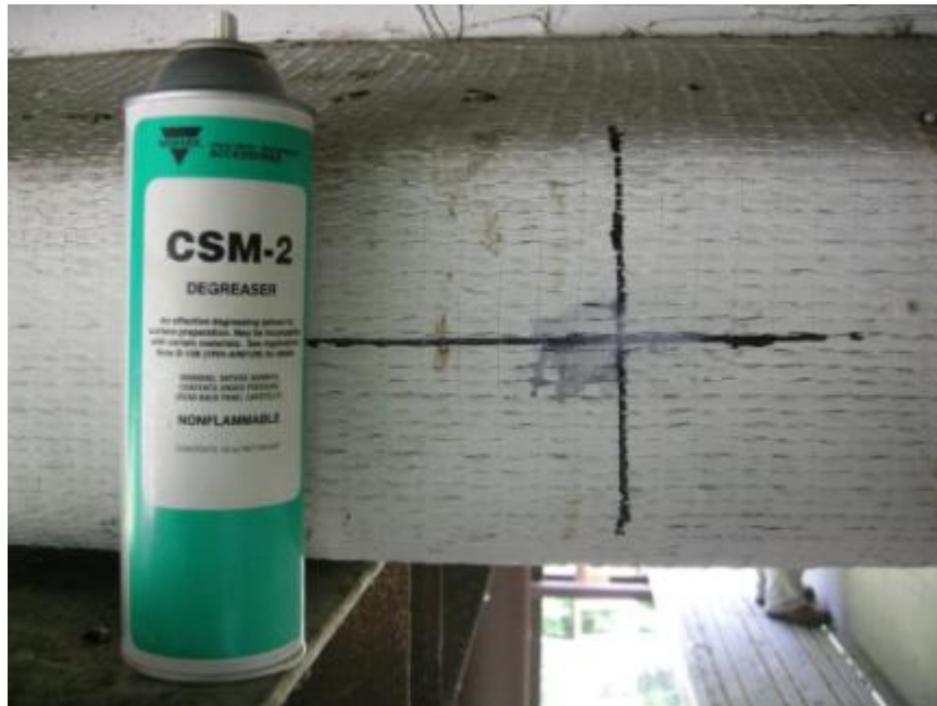
Figure 3.25: Strain gage installation—applying degreaser to gage location
