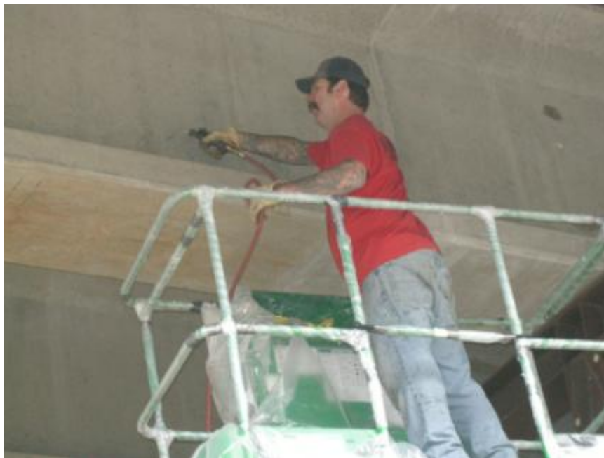
Figure 2.29: Surface cleaning—final removal of dust and debris
