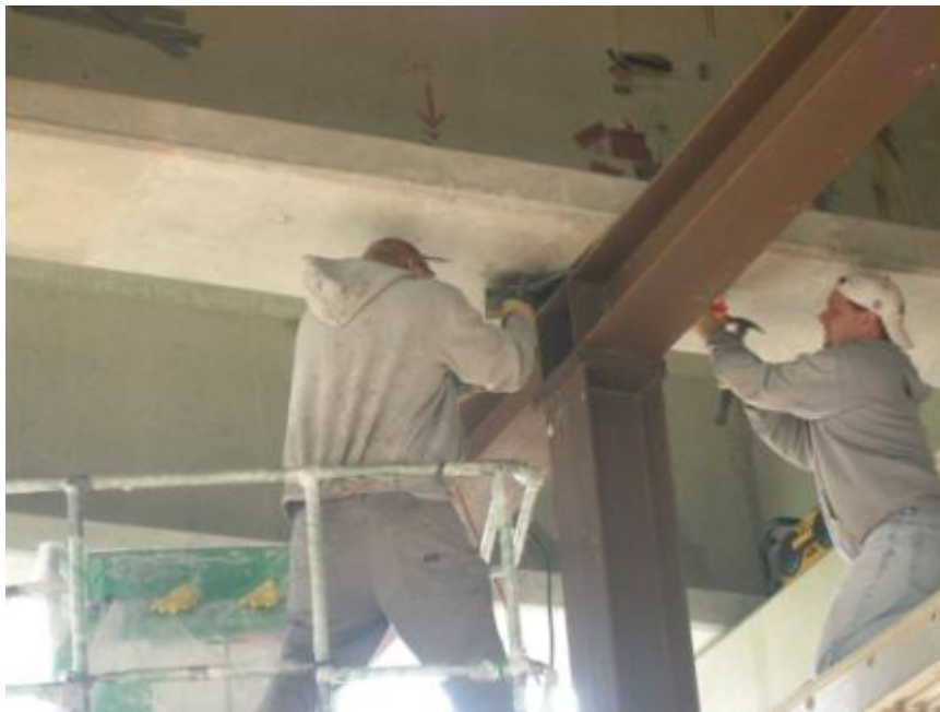
Figure 2.32: Successful removal of bearing pad
