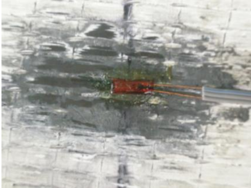
Figure 3.33: Strain gage installation—rubber coating for moisture protection
