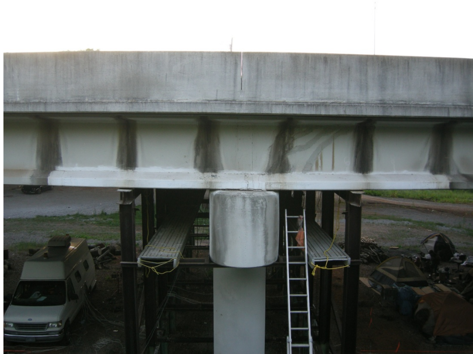
Figure 1.4: Girder 9 of Northbound Spans 10 and 11—repaired
