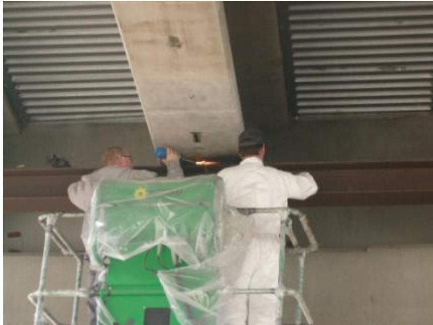
Figure 2.31: Use of torch for bearing pad removal
