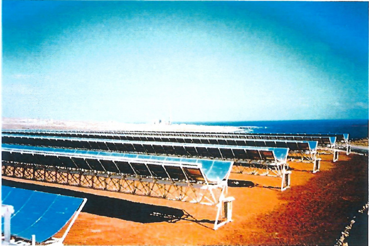
Figure 3.18 The Euclides 480 kW p system on the island of Tenerife (Spain) comprises a series of 14 linear parabolic trough mirrors 84m long (EPIA/BP Solar).
