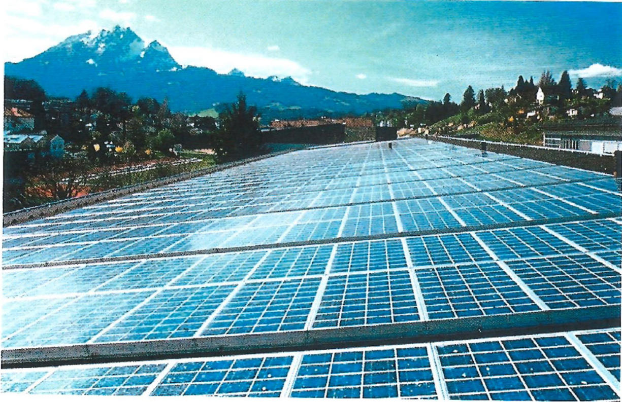
Figure 3.1 A large array of PV modules on a rooftop in Switzerland (EPIA/BP Solar).
