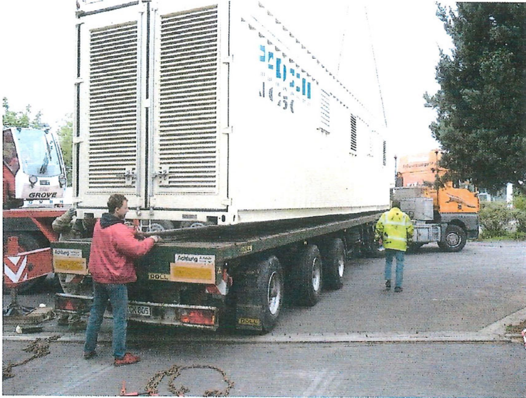
Figure 4.5 Scaling up: this 1.6MW p inverter weighs over 20 tons (Padcon GmbH).
