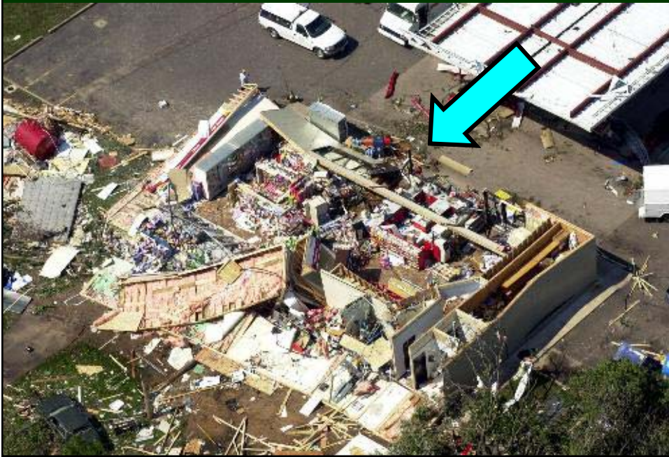
Wind damage from tornado
