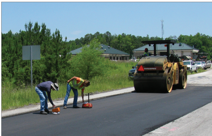
Monitoring field compactability on the NCAT Pavement Test Track
