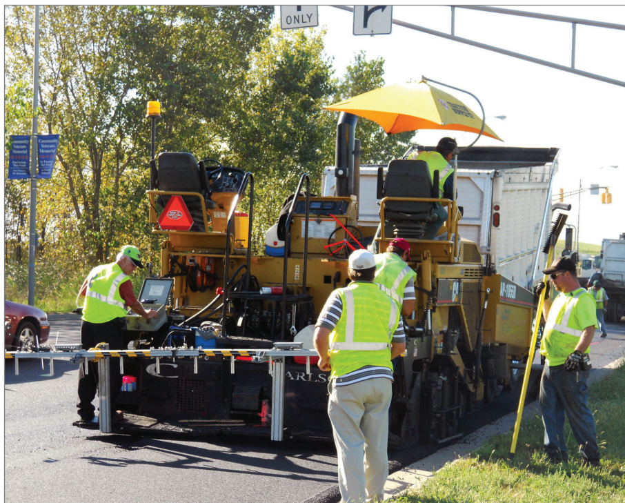
A warm-mix asphalt (WMA) placement job in Indiana
