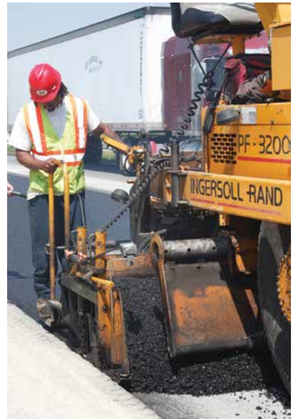
I-81 In-place pavement recycling project (Photo by Tom Saunders, VDOT)
