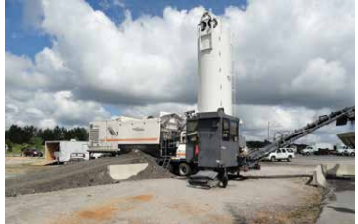
Figure 2 Mobile cold recycling mixing plant used during Test Track construction
