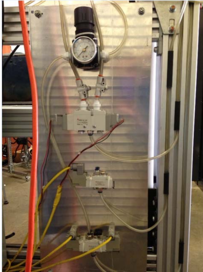
Figure 14: Valves and Pressure Regulator Mounted
